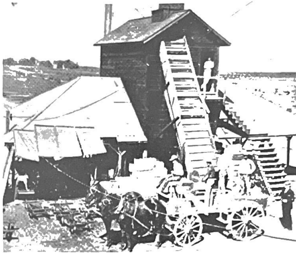
The West Side Fruit Growers Association, west of San Jose, had this fruit elevator next to its drying ground to convey the freshly dried prunes into its storage house.
