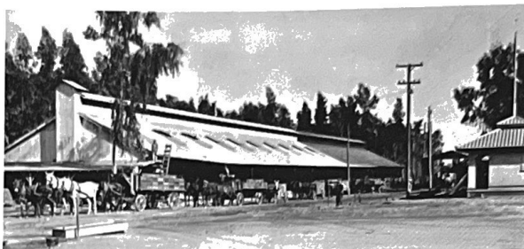
The concrete warehouse and packinghouse of the Mineral King Fruit Company, Visalia, in 1917, was 400 feet long and 80 feet wide, one of the fruit industry's largest.
